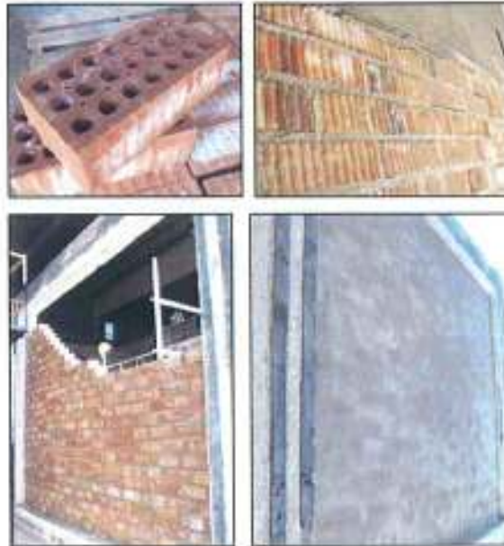
Images 3, 4, 5 and 6 – Details of the wall
