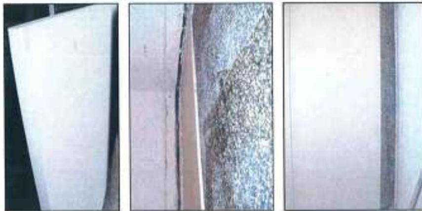
Images 9, 10 and 11 –Gypsum plasterboard is glued to the panel
