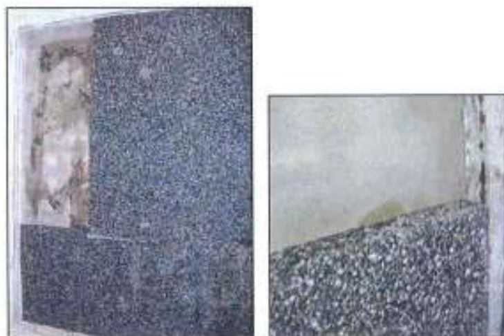
Images 7 and 8 – The panel is glued to the wall
